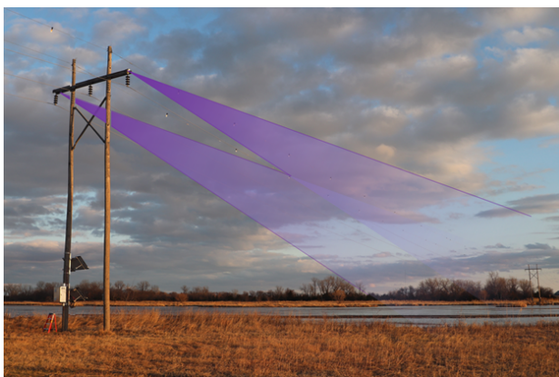
Fig. 2. Illustration of the Avian Collision Avoidance System's field of ultraviolet light illumination of power line crossings.
